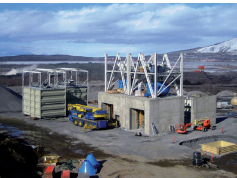
The Kiruna plant during erection, the 2 BHS 4.0 mixers in place.
