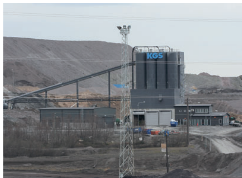
The new plant was designed by Röbäcks to operate at temperature below minus 30°C and in rough climate.
